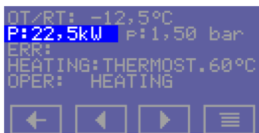
P: INST. POWER OF THE BOILER
