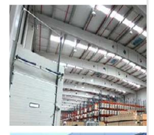
**Vertical Gas Air Curtains** - FACV series is specially designed to protect the building against uncontrolled external airflow through the doors. It helps to save energy which is used for keeping a desired temperature in the building. This series is made for vertical installation only.
